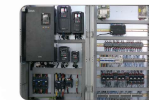
电器操控系统 Electric control system
